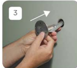
3 Insert anchor bar into wall
