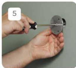
5 Tighten screw to secure anchor
